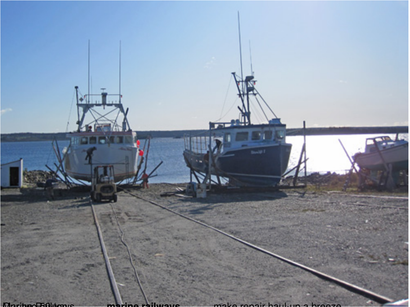
Marine Facilities marine railways make repair haul-up a breeze
